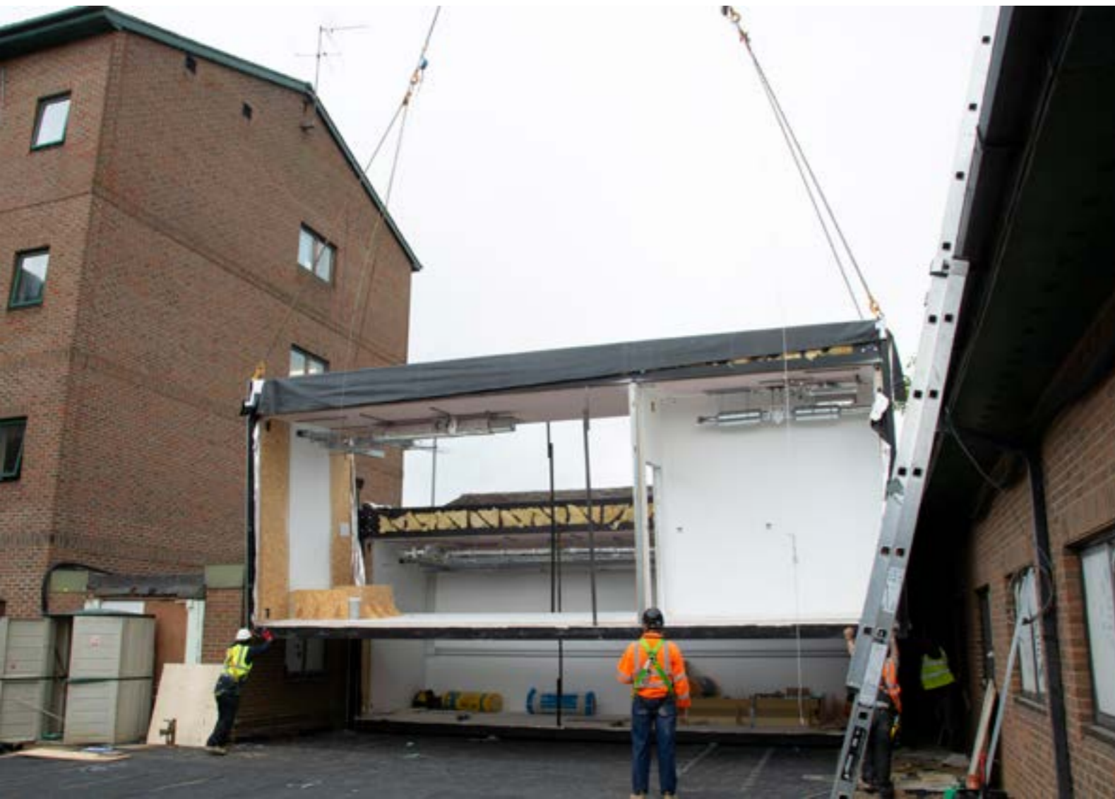
Construction of new emergency department
